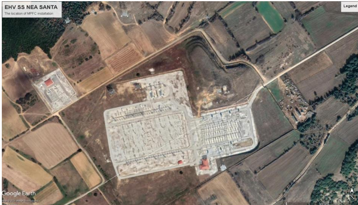
Figure 11: Top view of the Nea Santa Substation
